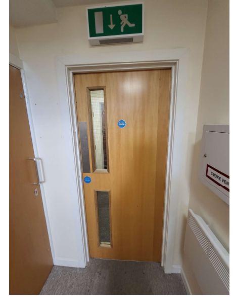
Internal Doors (Compartment Doors)
